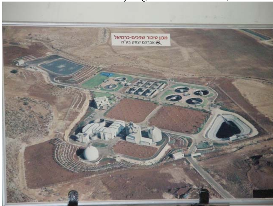
A photo of the WWTP - Karmiel
